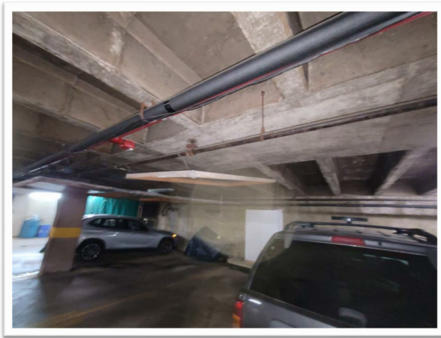
Figure 1.25 - Concrete beams and beam girders.
