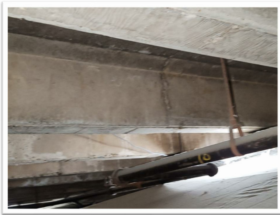
Figure 1.8 - Concrete Beam Girders over the plastic cover.
