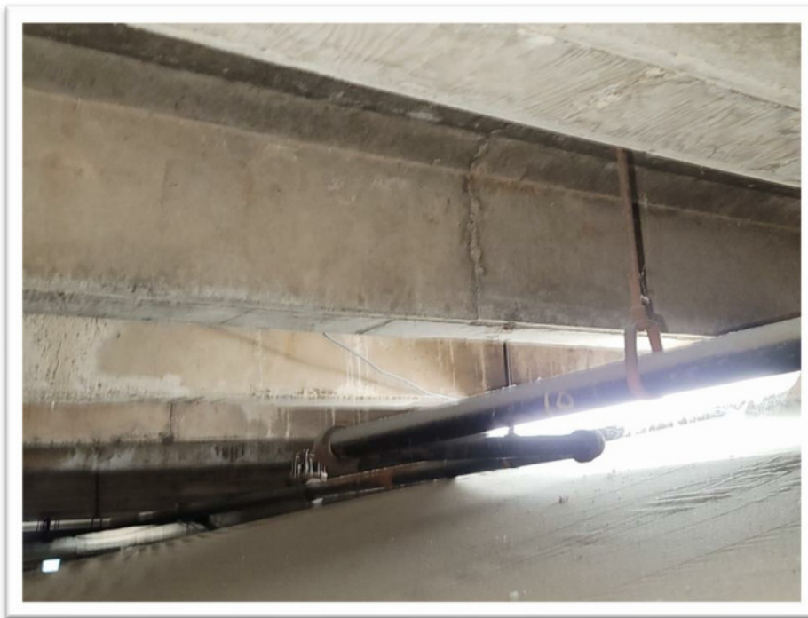
Figure 1.7 - Concrete Beam Girders.
