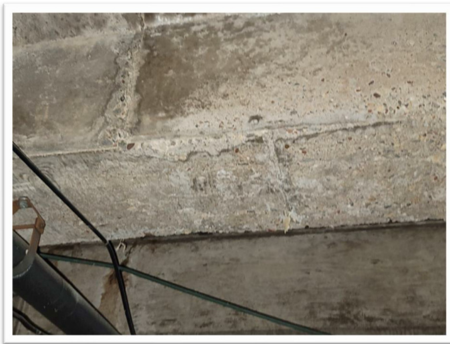
Figure 1.5 - Concrete Beam Girders.
