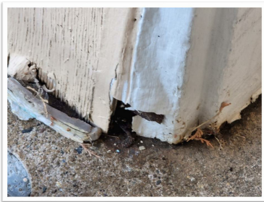
Figure 3.43 - Rot damage.
