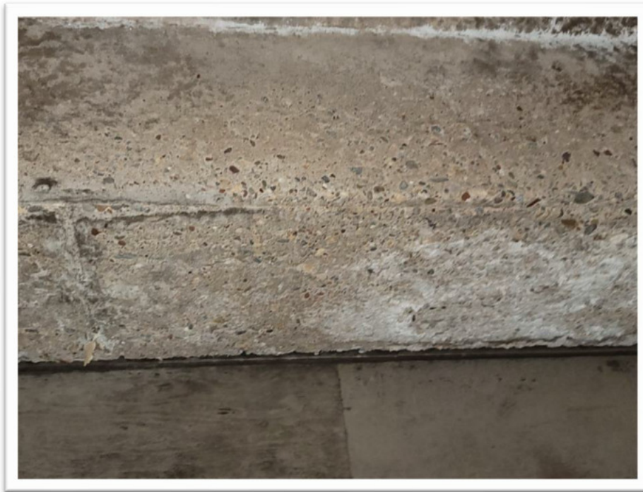
Figure 1.6 - Concrete Beam Girders.
